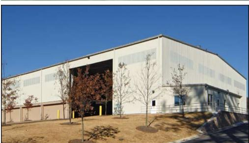
Translucent Wallites provide natural diffused light for brighter working conditions with the potential to save energy and lighting costs. Wallites are available in Panel Rib and Vee Rib wall profiles.
